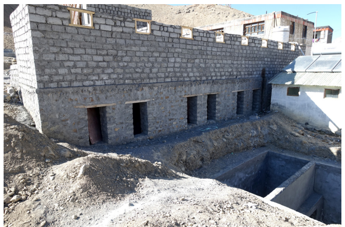
The new dual function toilets being built at Munsel-ling are both water-septic and composting
