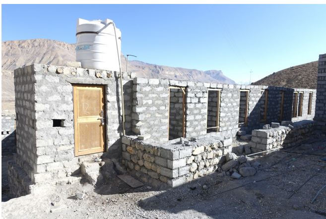
The new dual function toilets being built at Munsel-ling are both water-septic and composting
