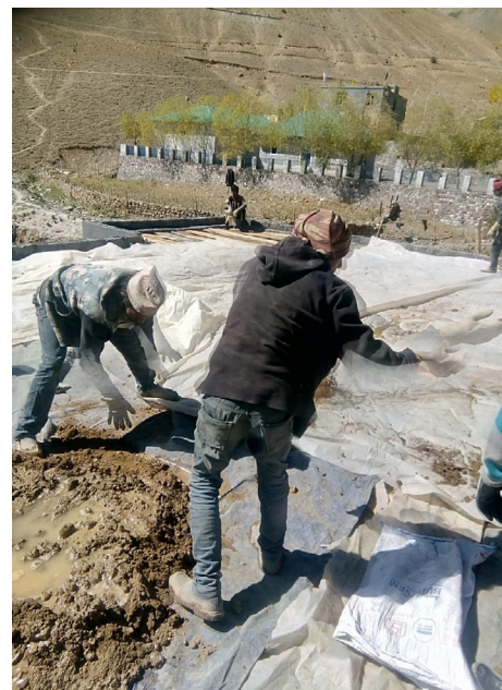
Workers applying a weatherproof layer to earthen roofs.
